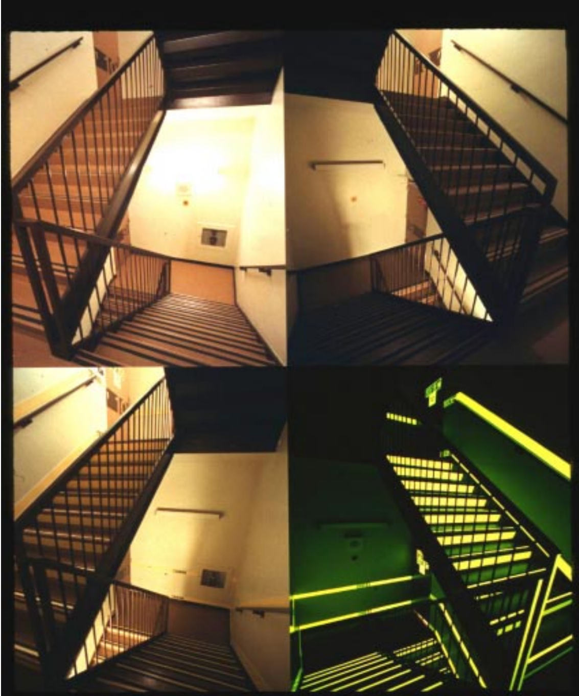
Figure 3: Pictures of the Four Stairwells
